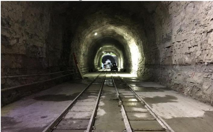
The tunnel is being excavated by a Tunnel Boring Machine (TBM) like the one shown in the photo to the right. These machines are designed to bore through the limestone, creating the 21.5 foot diameter opening. The rock material is hauled out and away through the shafts, and then the tunnel is lined with cast-in-place concrete resulting in a circular tunnel with a 19 foot inside diameter.
