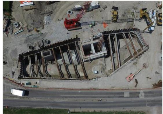
Shaft drilling work for all of the intake structures was completed in spring 2017. As of July 1, 2018: construction of the Chain of Rocks Drive intake is 75% complete with work continuing through fall 2018; construction of the Church Drive intake is 6% complete with work continuing through summer 2019; and construction of the CSO 052 intake is 95% complete. Construction of the pump station will continue through fall 2020.
