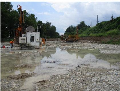
Installation of the secant pile wall began in December 2017 and includes 78 secant piles extended into the top of bedrock. This work was about 15% complete as of January 1, 2018.
